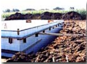
A typical TF foundation set up, braced and ready for pouring.
