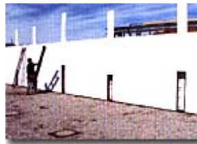
An important feature of the TF System™ is the ability to raise & lower panels
